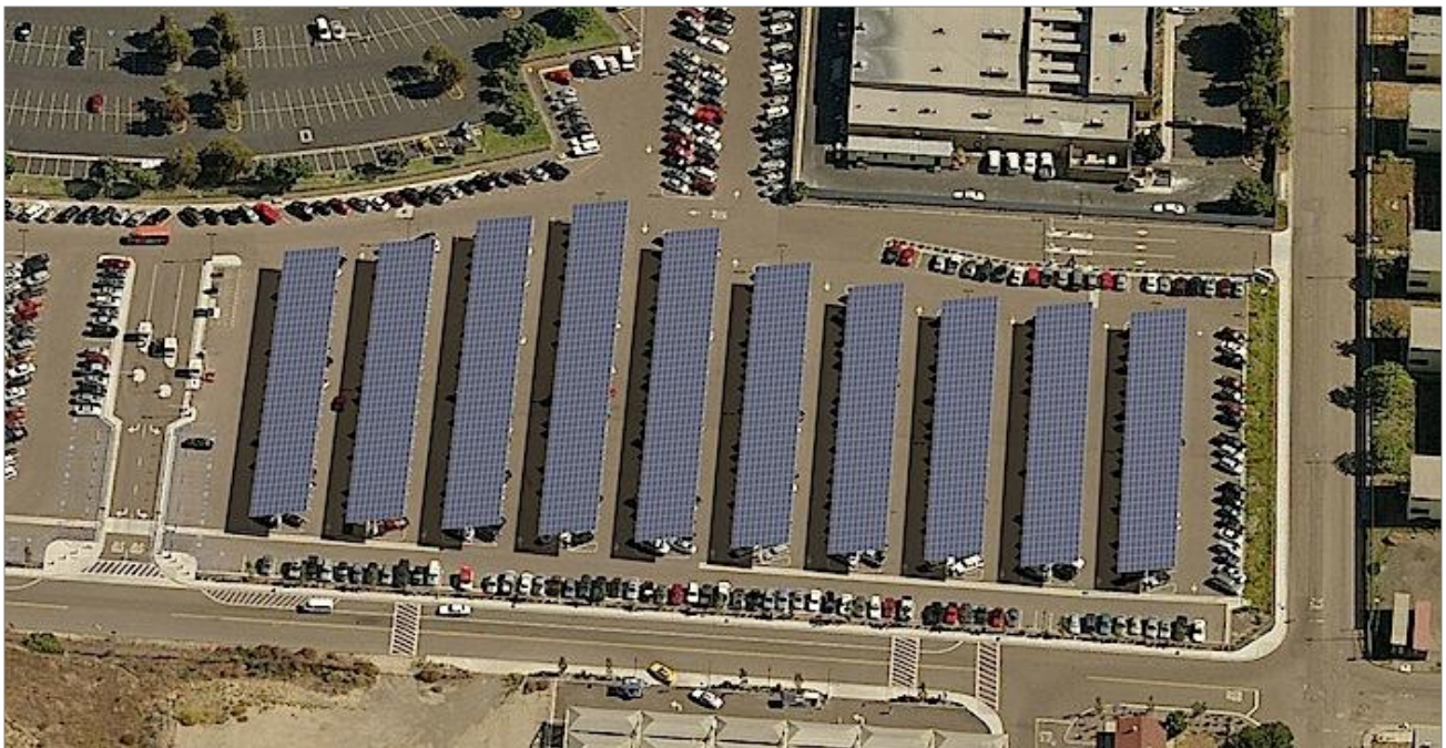
New Solar Panels at the San Diego International Airport
